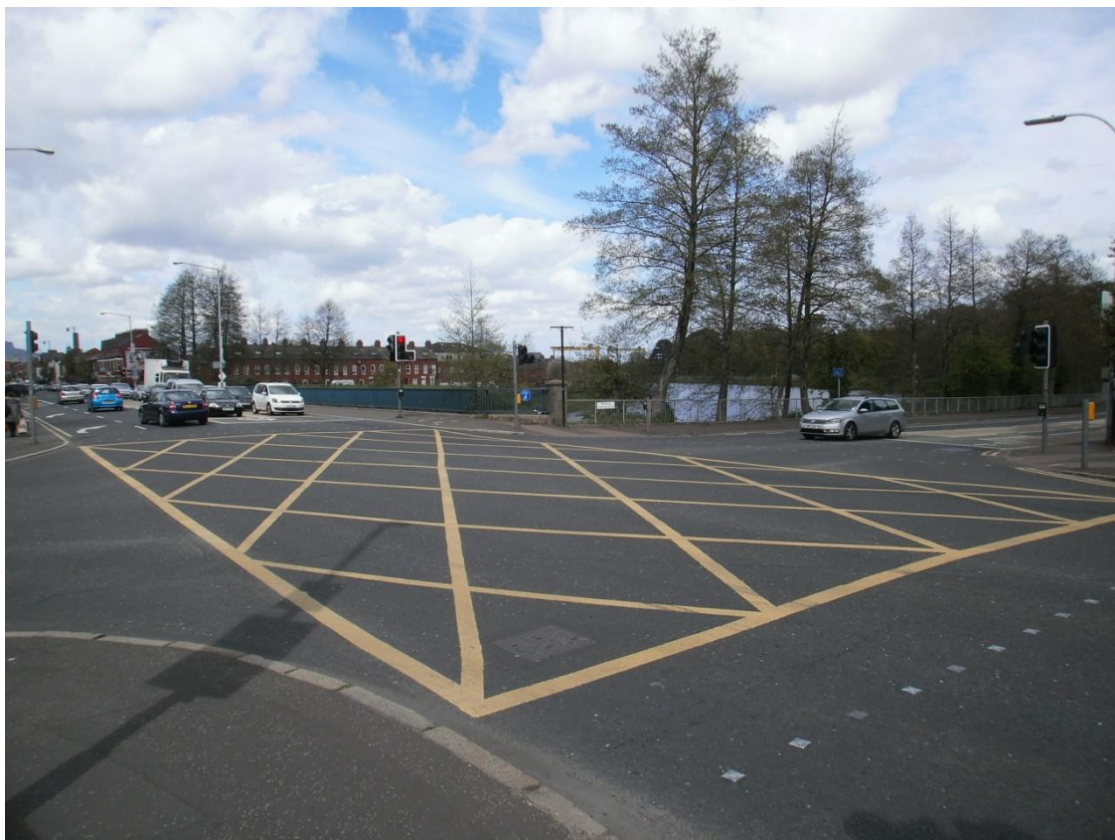
Ormeau Road at Annadale Embankment – yellow box junction marking
